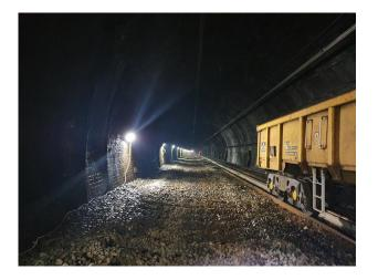
In addition to monitoring the tunnel lining, track monitoring was also conducted. This used a total of 834 Senceive High-G Triaxial Tilt Sensor Nodes at 3 metre intervals throughout the main works area and 30 m beyond the zone of influence. Relative and absolute twist and cant were monitored. The absolute cant was calculated using surveyed cant readings, which was then used as a constant offset to the incoming data from these tilt sensors.
